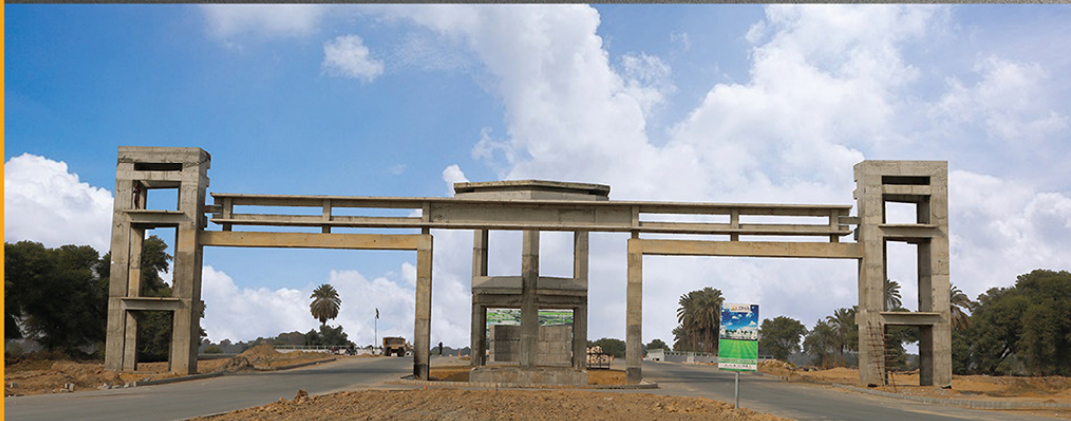
DEVELOPMENT WORK AT DHA BWP MAIN GATE
